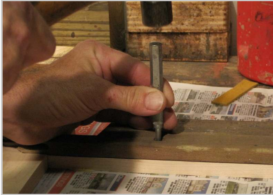
Photo 349: The location for the screws holding the back rail to the keybed are marked using the old back rail as a template.
