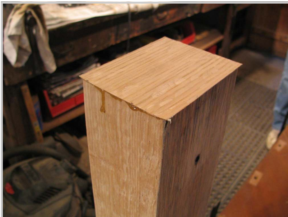
Photo 140: The last piece to go on is the front, which overlaps the top and the sides, as was done originally. This piece is intentionally cut a bit large. It will be sanded down flush once the glue is set.
