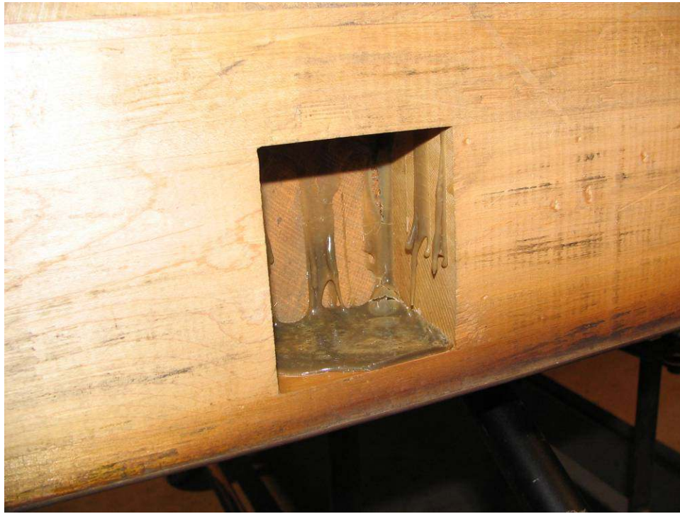
Photo 17: You can still see the bubbles in the glue!
