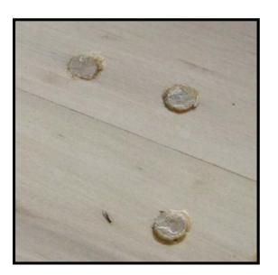
**Step 24:** Allow the glue to set for at least an hour or two before proceeding.
