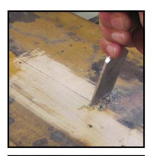
Step 7: To refinish the bottom board (if that step seems necessary) first remove the old finish by scraping with a chisel. The most effective method is to bear down on the chisel as you drag it towards you over the old finish. The beveled edge of the chisel should be away from you, while the blade is tipped slightly in towards you as shown.
