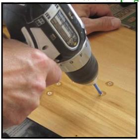
**Step 32:** For brackets and trapwork mounts which are to go back to the same location as they were originally found, drill the appropriate size of pilot hole for each screw. (These screw holes are being drilled on a diagonal to match the original slant of the screws.)
