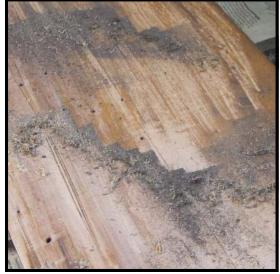
**Step 8:** Continue scraping until the bulk of the old finish has been removed. While chemical strippers may be used for this step, using a chisel to do the job is usually pretty simple, in that the old finish is often shellac and is easily scraped off.
