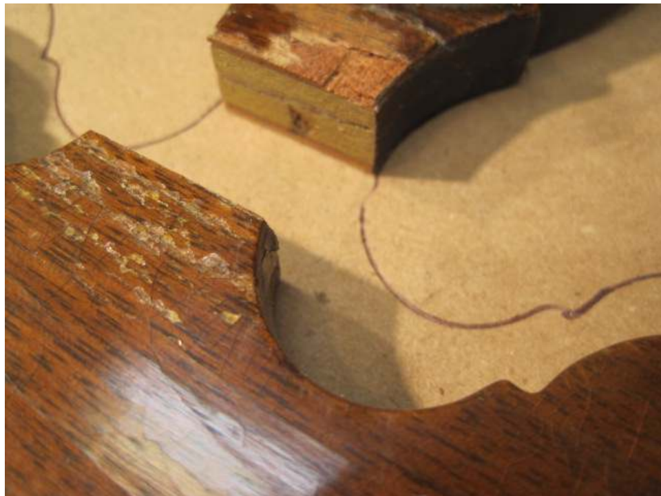
Photo 27: Now, by using the paper pattern, the exact width of core wood needed to fill in for the missing wood can be determined..
