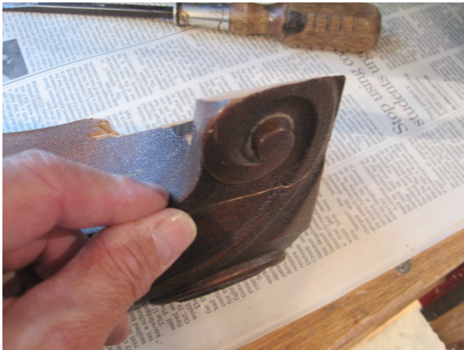
Photo 2: The first step is to glue the smaller chunk and let it set overnight.
