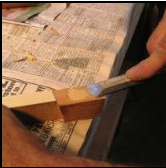
**Step 19:** For small gouges and divots, a commercial wood filler will do the job. Apply with a little overfill, and allow to dry completely.
