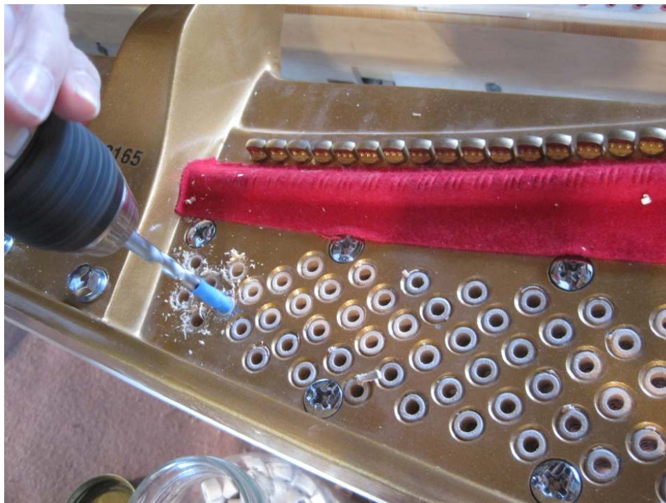
Photo 89: Each bushing is reamed to allow for the tuning pins.
