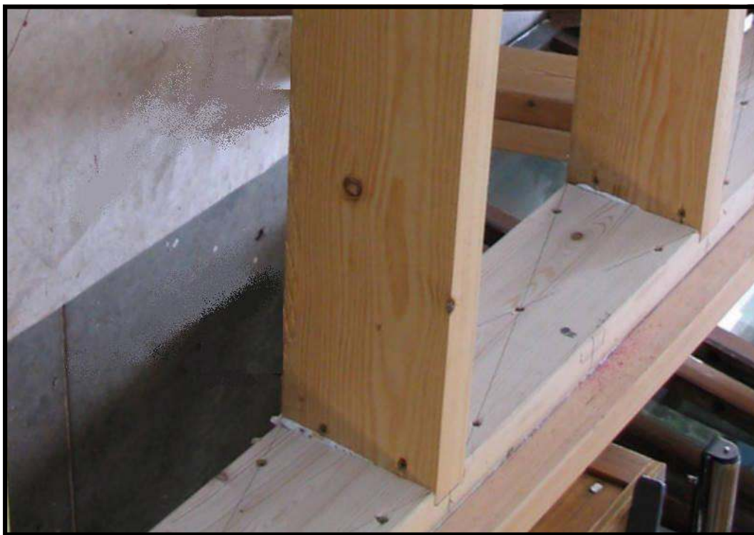
Inner frame and outer frame are screwed and glued together.
