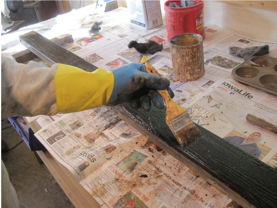
Photo 14: First heavy coat of stripper is applied.
