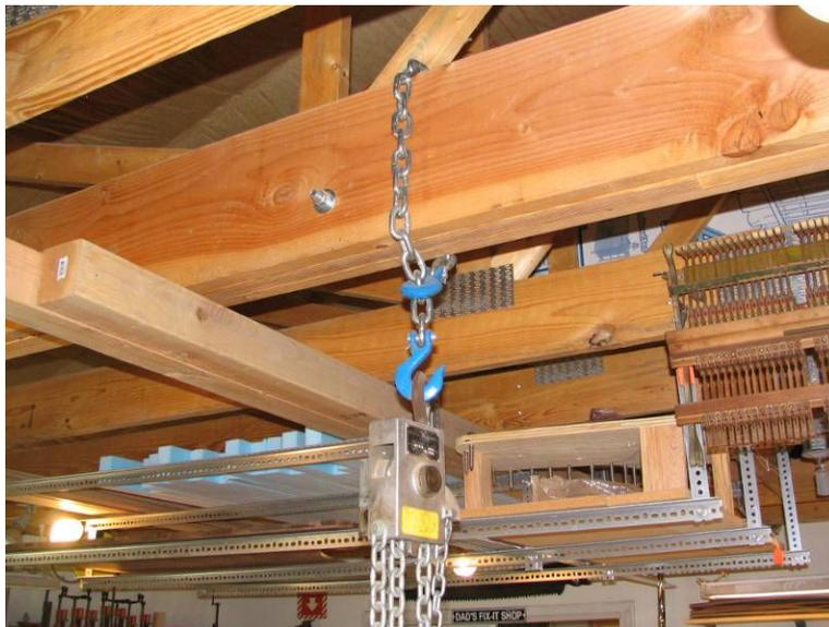
*Photo #7: Solid support for a hoist is essential*
