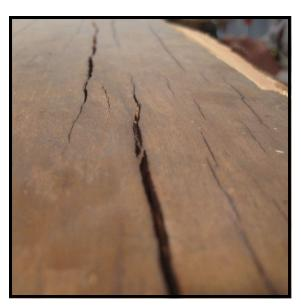
With such a covering in place, it is impossible to see the extent of the separation, let alone deal with repairing it. In the case of the maple cap glued in place in the photo to the left, the fissures which had opened up in the cap gave evidence of the separation occurring below it, but until the cap was removed, nothing could be done.
