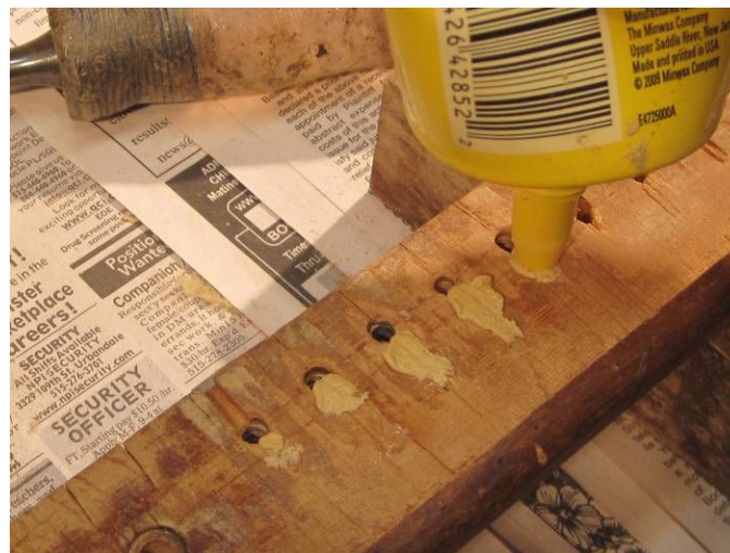
Photo 7: Repairing the damage.
