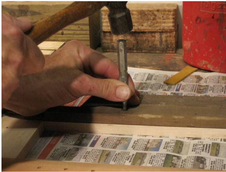
Photo 4: Using the old back rail as a template.
