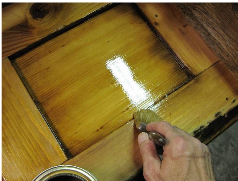
Photo 7: A clear coat to form an odor barrier.
