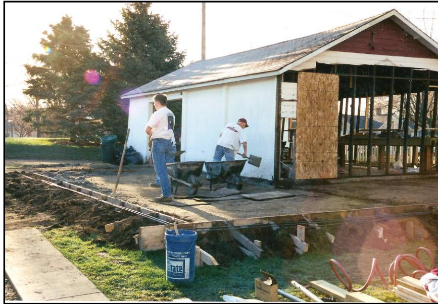
Photo 3: Adding floor space.
