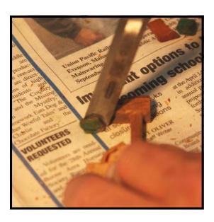
Step 4: With the flat edge of your 1/2" chisel up against the underside of the catcher, shave off the catcher felt. A pivoting motion, with the corner of the chisel against the bench, works best. The chisel must be sharp for this operation and even so, there may be felt and glue residue which remains. Be cautious not to remove wood from the catcher in the process. You will clean up any residue with a file in a later step.
