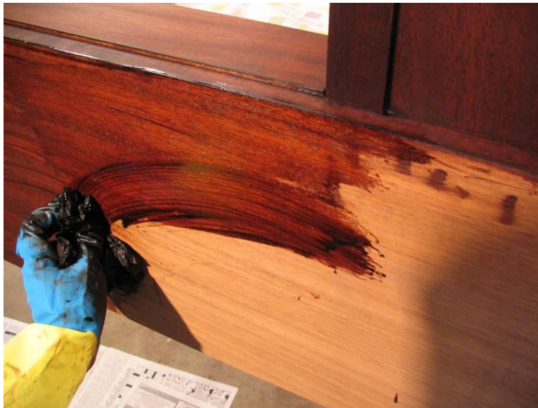
Photo #2: Stain is applied
