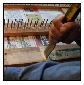
**Step 7:** Scrape off the remains of the old glue and felt using a wide chisel, pulling it towards you as shown. If you try pushing the chisel away from you, it's easy to gouge the wood.
