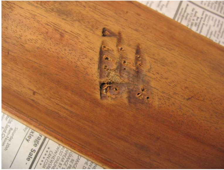
Photo 4: Badly damaged fallboard with anchor holes drilled
