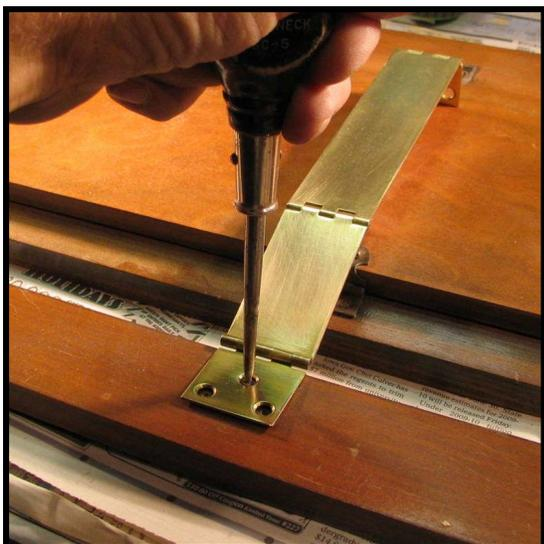
**Step 4:** With the hinge in position, mark the screw holes with a sharp awl.
