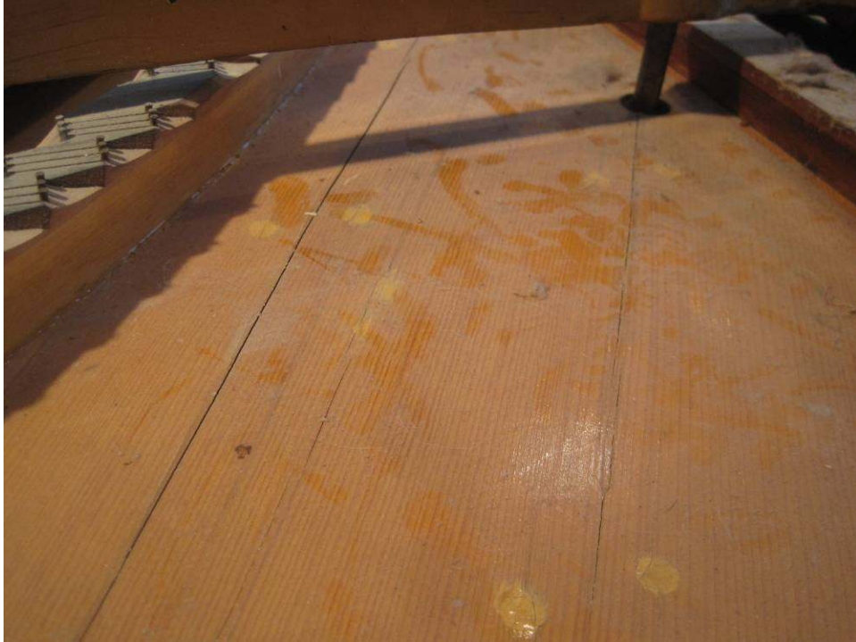
Photo 19: Grand soundboards are very hard to clean when the strings are in place. Typically, the grime just has to stay there. With the strings out of the way, this odor-holding layer of dust can be properly cleaned up.
