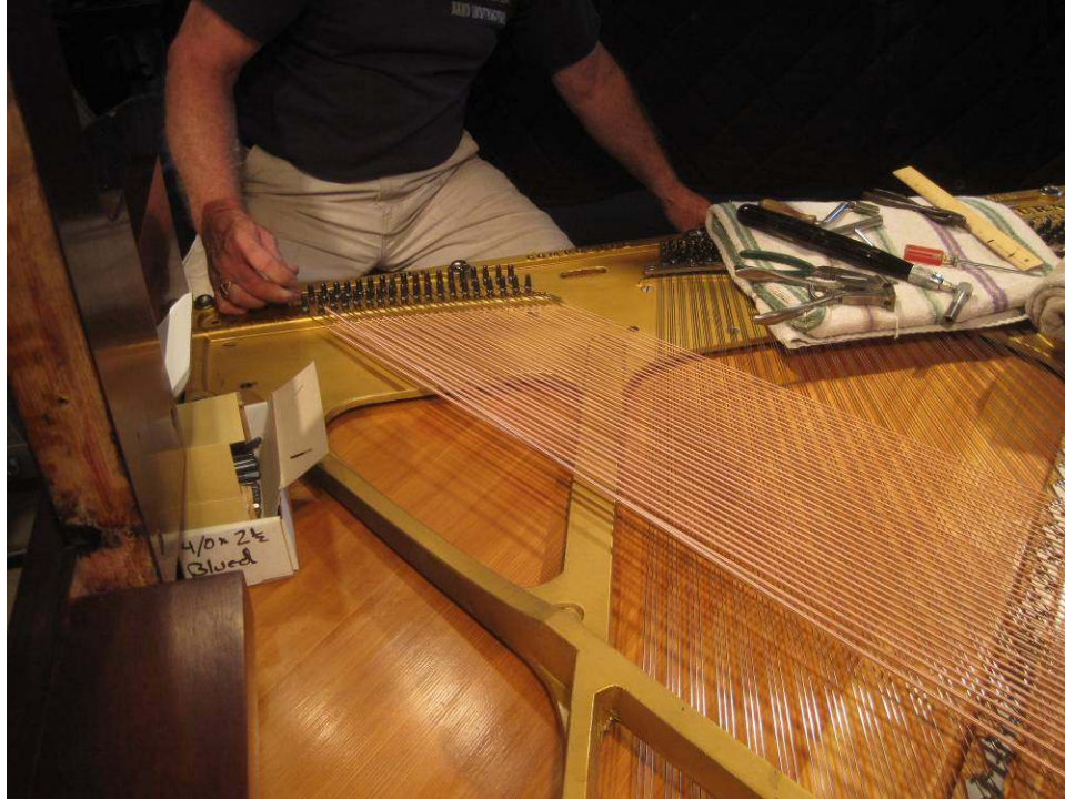
Photo 93: With the plate bolted back into place, Dave works on restringing and repinning the piano.
