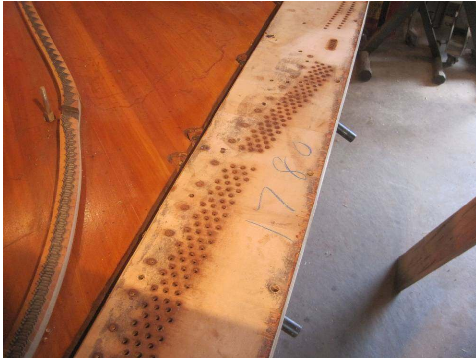
Photo 17: The pinblock is in excellent condition. No sign of chemical treatment that would make repinning less effective.
