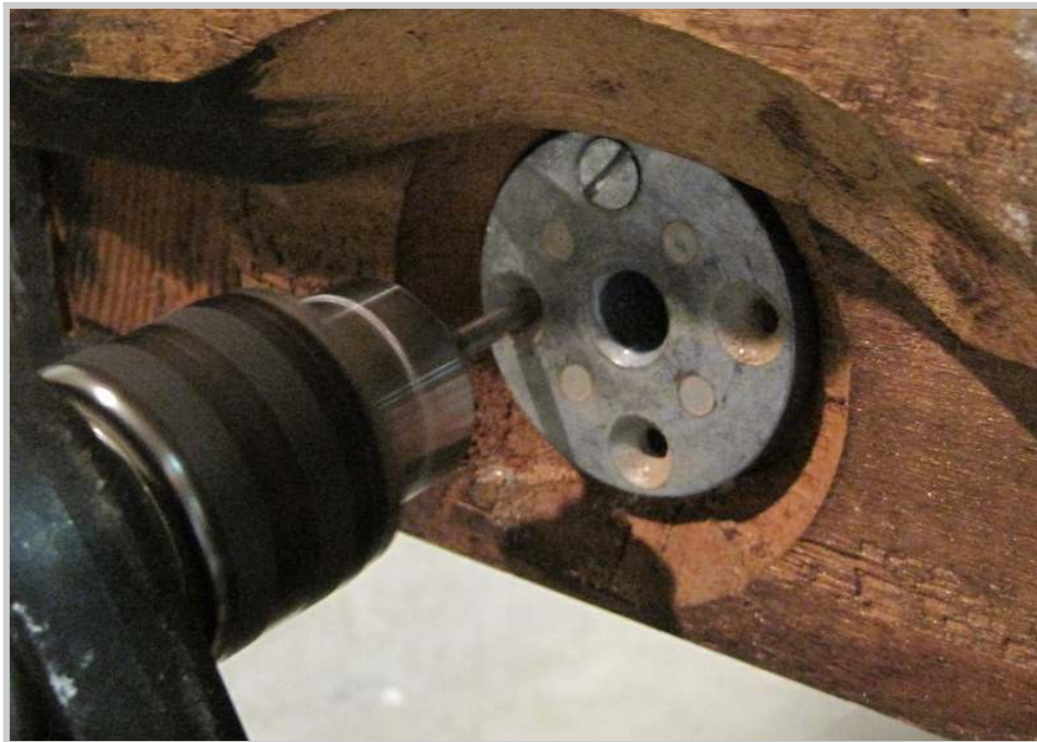
Photo 309: New sockets for the new casters are added in.. . .
