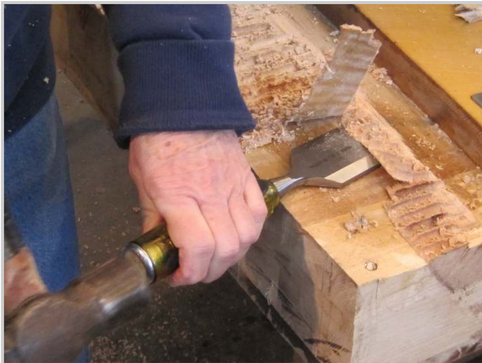
Photo 137: Bev works away at the job with the hammer and chisel. With the steam and heat, the remaining layer of pinblock material begins to come off. Although we weren't able to finish the job on this day, we made considerable headway - on our next work day we should have the surface completely prepared for the new pinblock.
