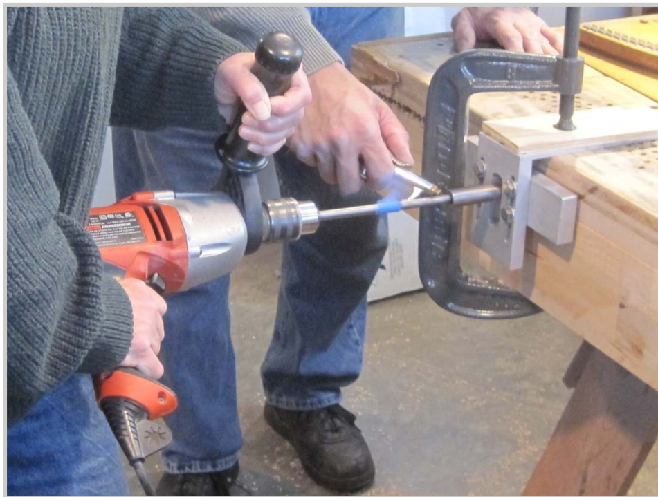
Photo 105: As the drilling progresses, chapter members switch off to give everyone a chance to try out the process. The blue tape on the bit marks the depth of the hole to be drilled.
