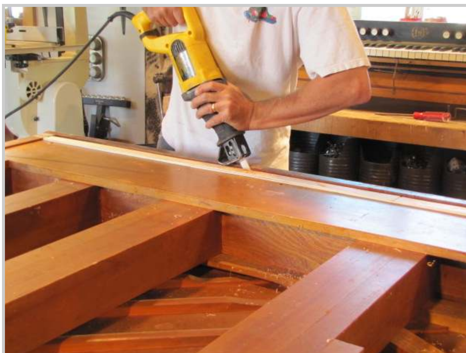
Photo 73: A final quick pass with a reciprocating saw completes the job.
