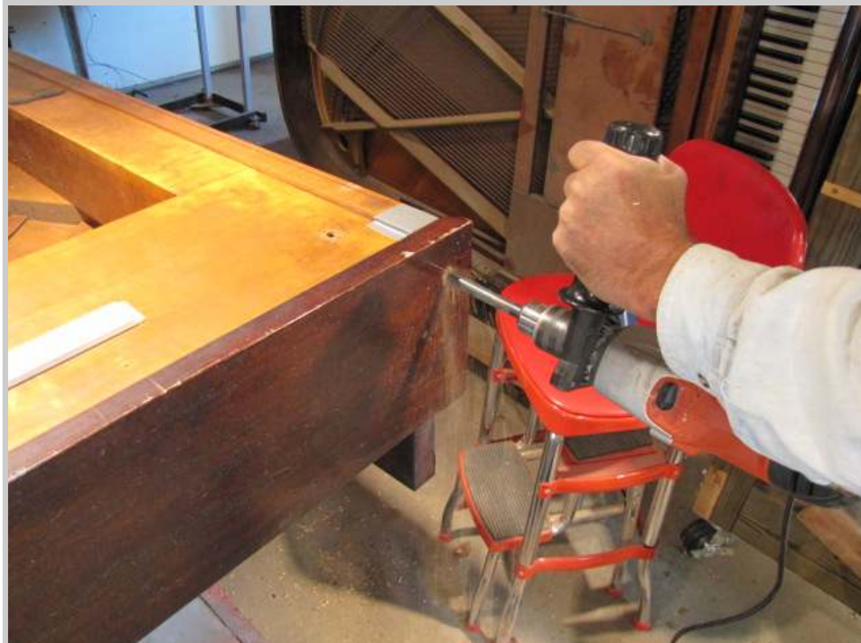
Photo 66: Likewise with the top. These holes will be doweled when things go back together, and covered with plugs cut from mahogany veneer. After refinishing, they will be practically invisible.
