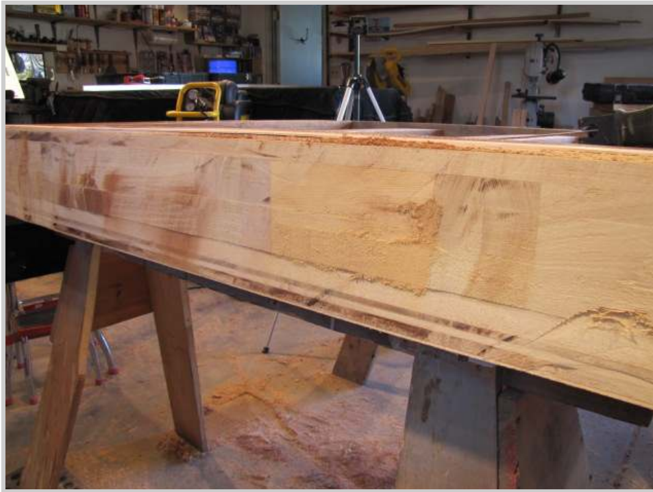
Photo 74: The exposed wood of the frame and pinblock. The wood is a bit uneven from the sawing process.
