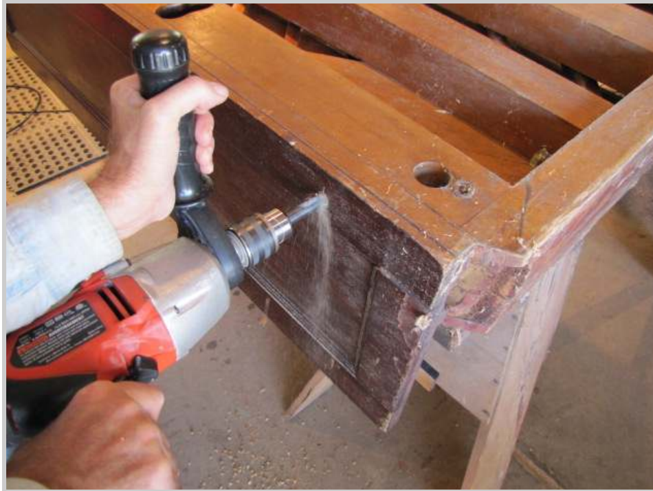
Photo 65: Two 1/2" indexing holes are drilled in either side to facilitate replacement of the sides at the exact location from which they are removed.
