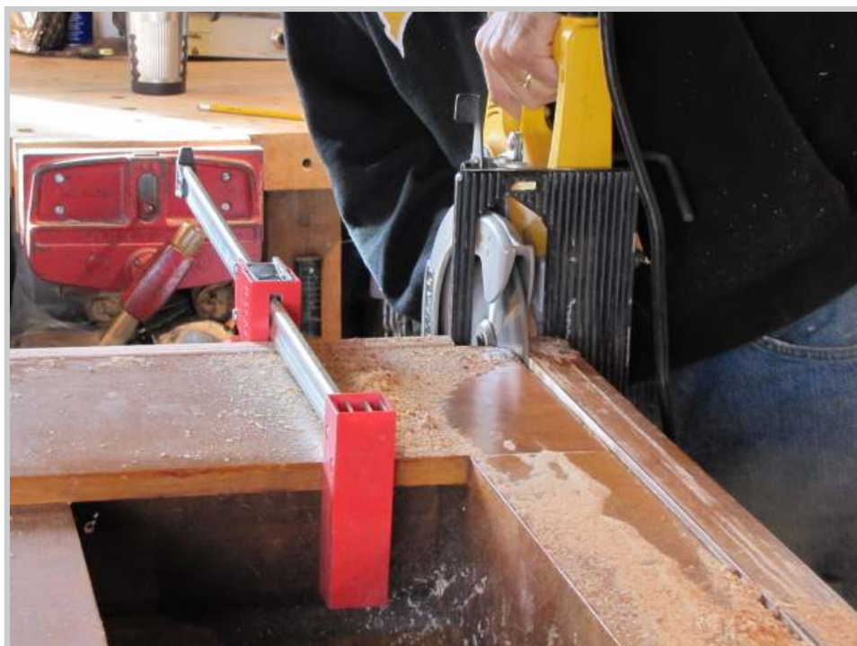
Photo 77: Using a smaller, easier to handle saw, the cut is extended around the corner.
