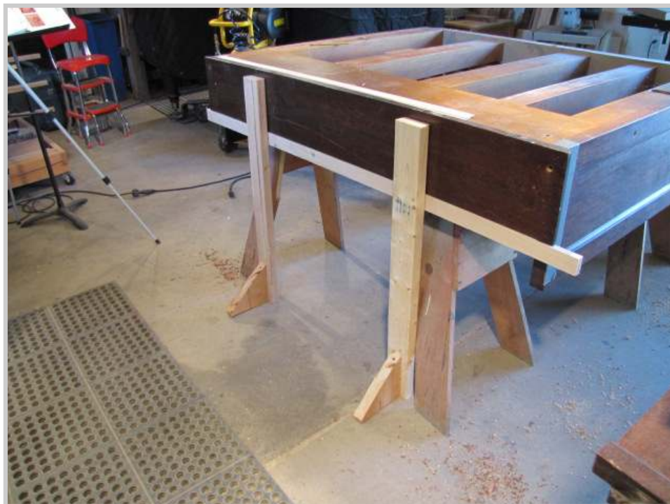
Photo 69: To prevent the top from falling and being damaged, a set of 2 X 4's with a crossbar is constructed to catch the top when it is freed.
