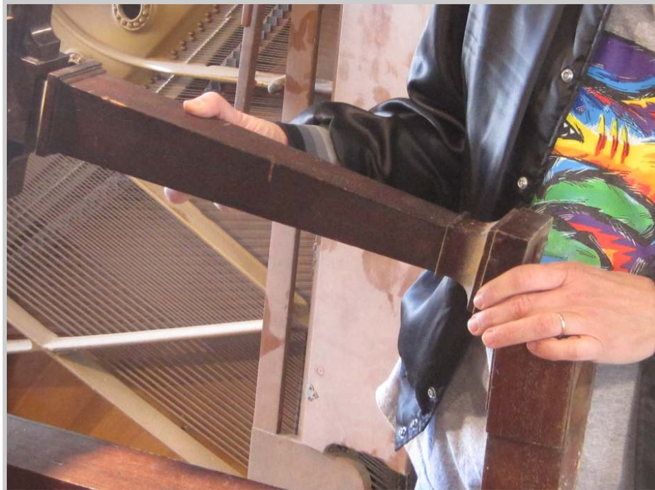
Photo 18: Steve removes two small bracket screws and the legs easily slide off.
