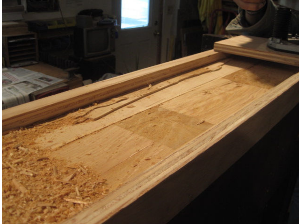
Photo 14: This works much better than the chisel. I take off 1/8" at a time, and get down to the source of the problem.
