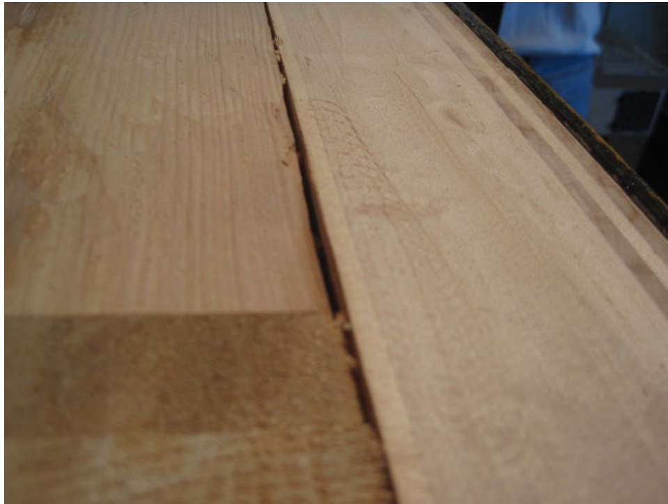
Photo 15: A separation of glue joints from one side to the other will require attention. When the strings and pins have been removed, we will glue, clamp and bolt the back together before putting on a new maple cap.
