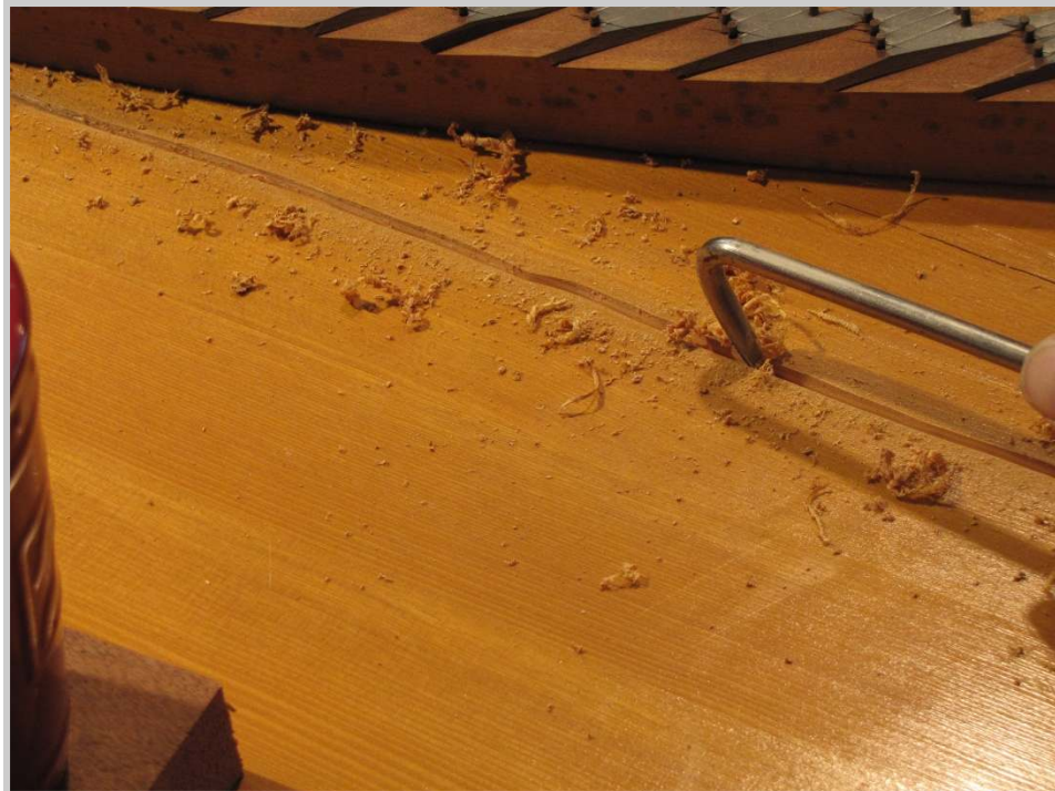
Photo 47: Each crack is widened with a specialized gouging tool which produces a v-shaped gouge suitable for shimming. Multiple passes with the gouging tool with a moderate amount of downward pressure produce the cleanest cut.
