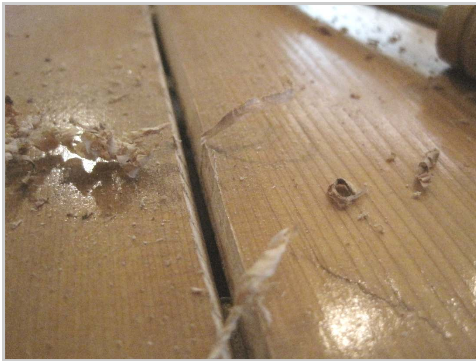
Photo 48: A perfectly gouged channel for a shim.
