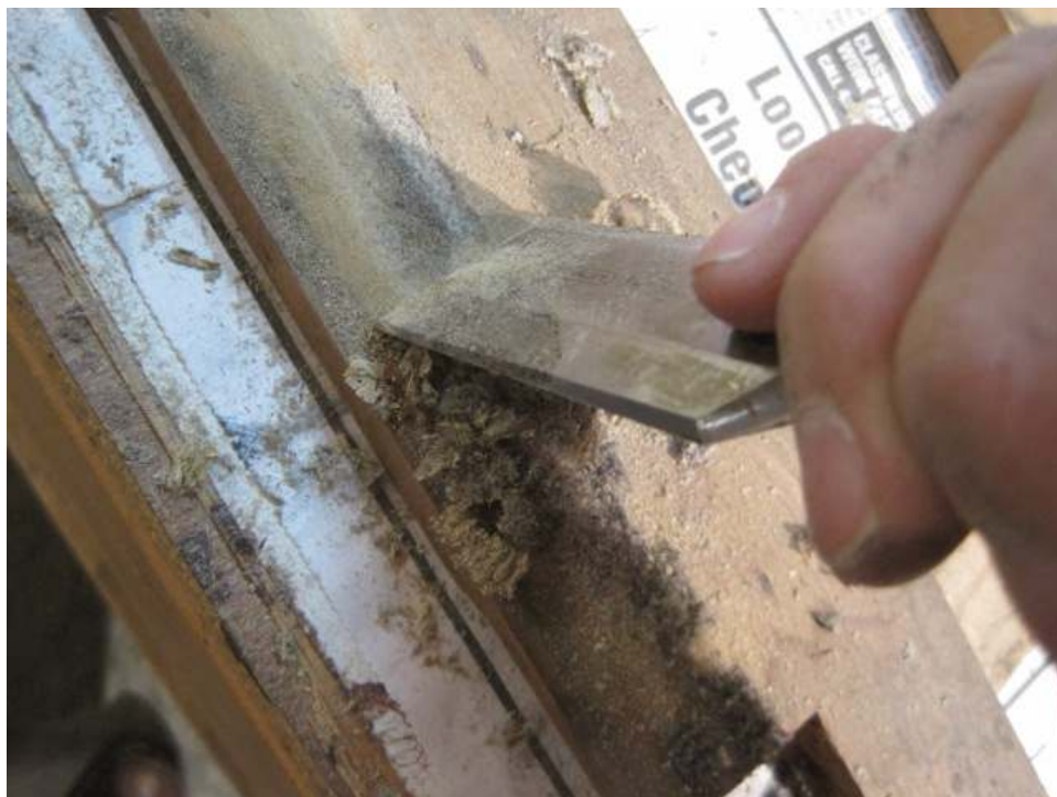
Photo 74: A sharp chisel is then used to scrape off excess glue and felt.
