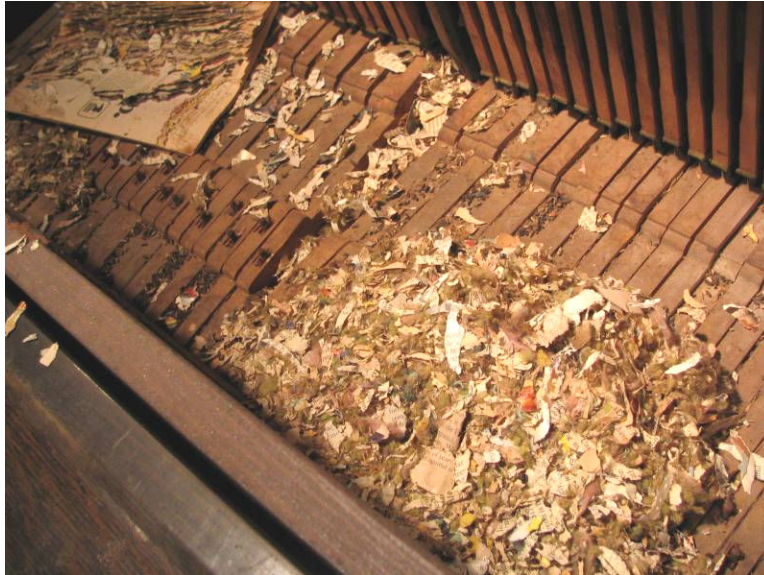
Photo 2: Would you want to dig down under this mess?
