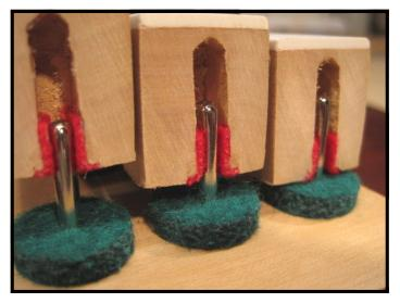
Smooth, polished keypins and good quality bushing felt (the red felts on the insides of the mortises, shown in the above cut -away photo) are essential for this system to work efficiently. By carefully removing the old pins and replace them with a new set of high-quality keypins, the touch of your piano will be improved.
