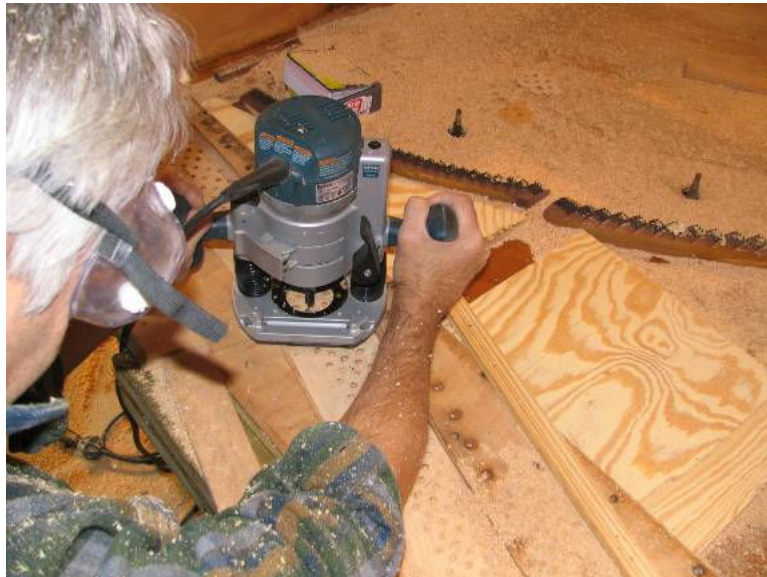
Photo 4: Deepening the cut
